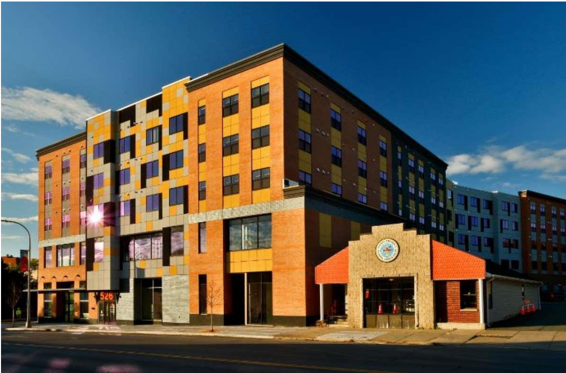
The Swinburne apartment mixed use building on Central Avenue, Albany, is complete. Courtesy HCR
